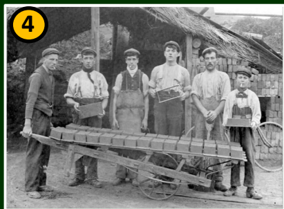
Brickies mixed cinder dust with the clay bricks(4) and baked them in the kilns (5)
