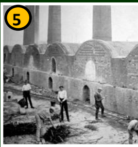
Brickies mixed cinder dust with the clay bricks(4) and baked them in the kilns (5)
